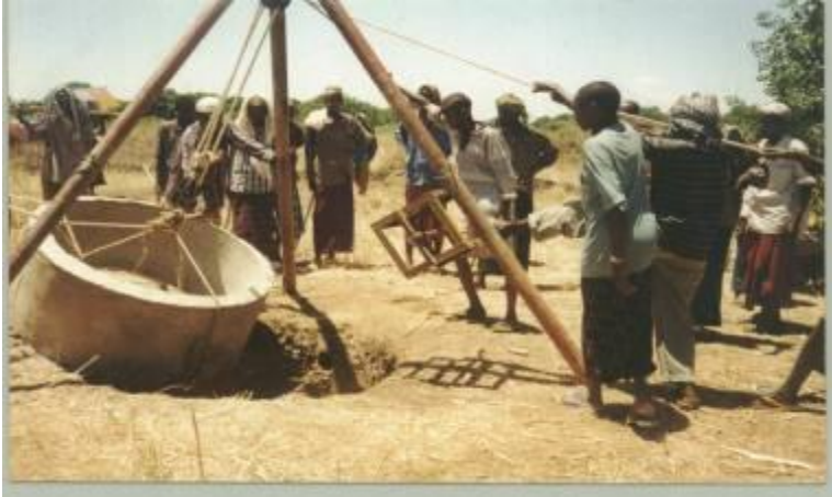
Construction of shallow wells at Abalatiro
